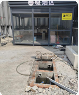
Floor Washing Water Three-Stage Sedimentation Tank
